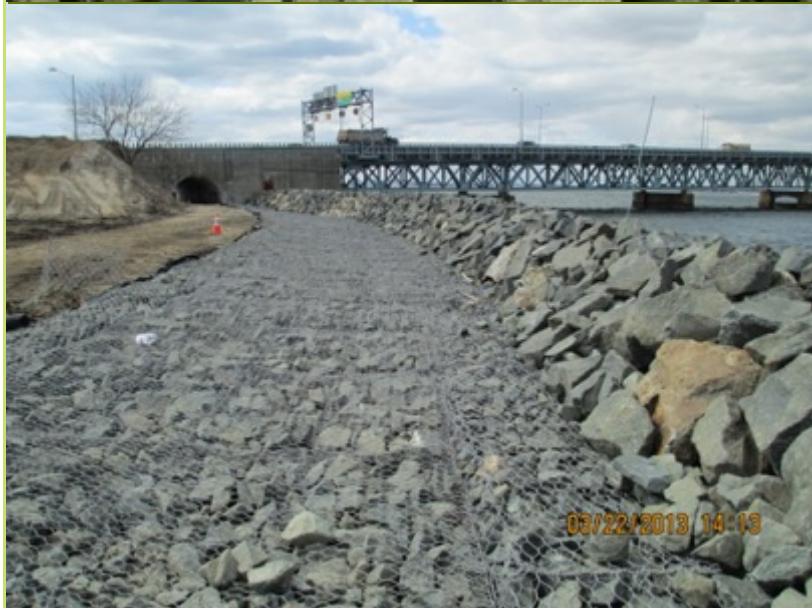
Restored abutment at Cross Bay Bridge
