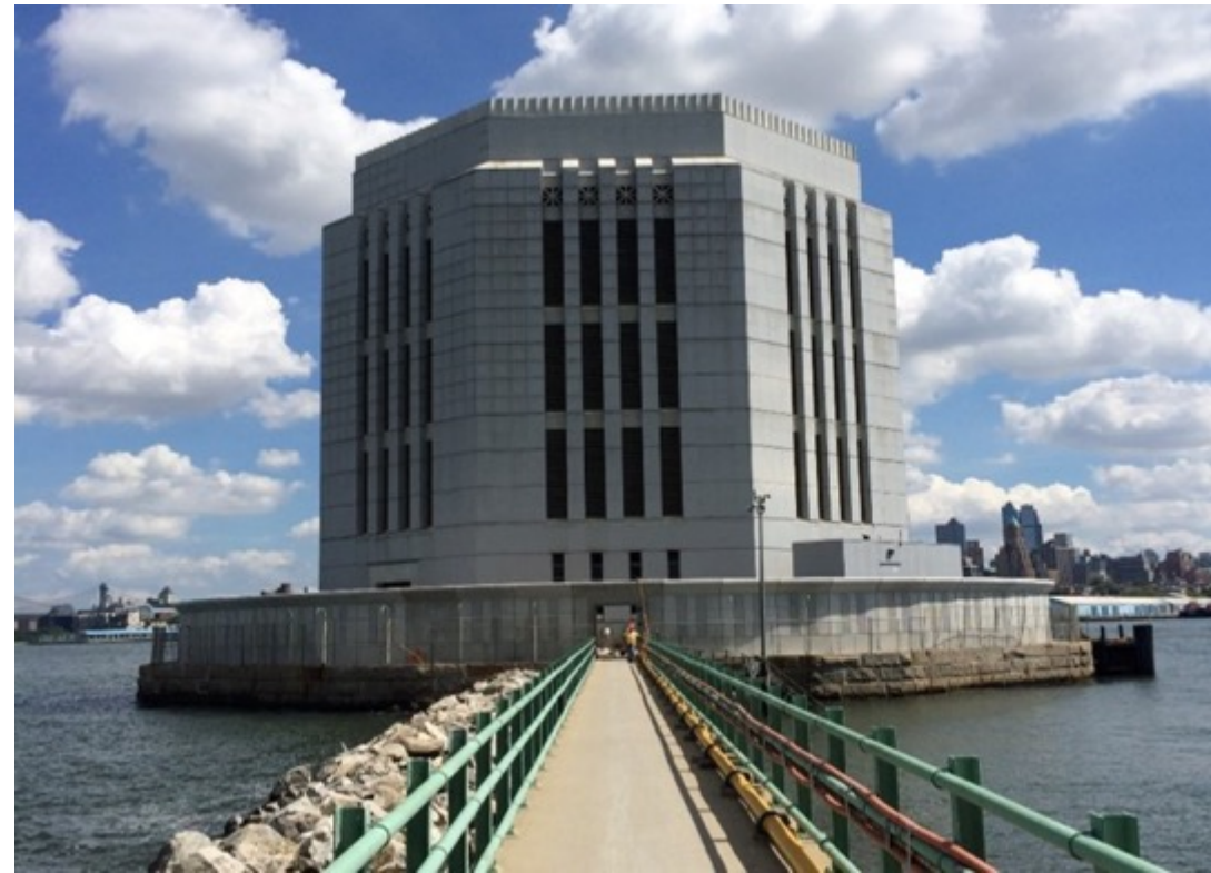
Sea Wall at Gov. Is Ventilation Bldg
