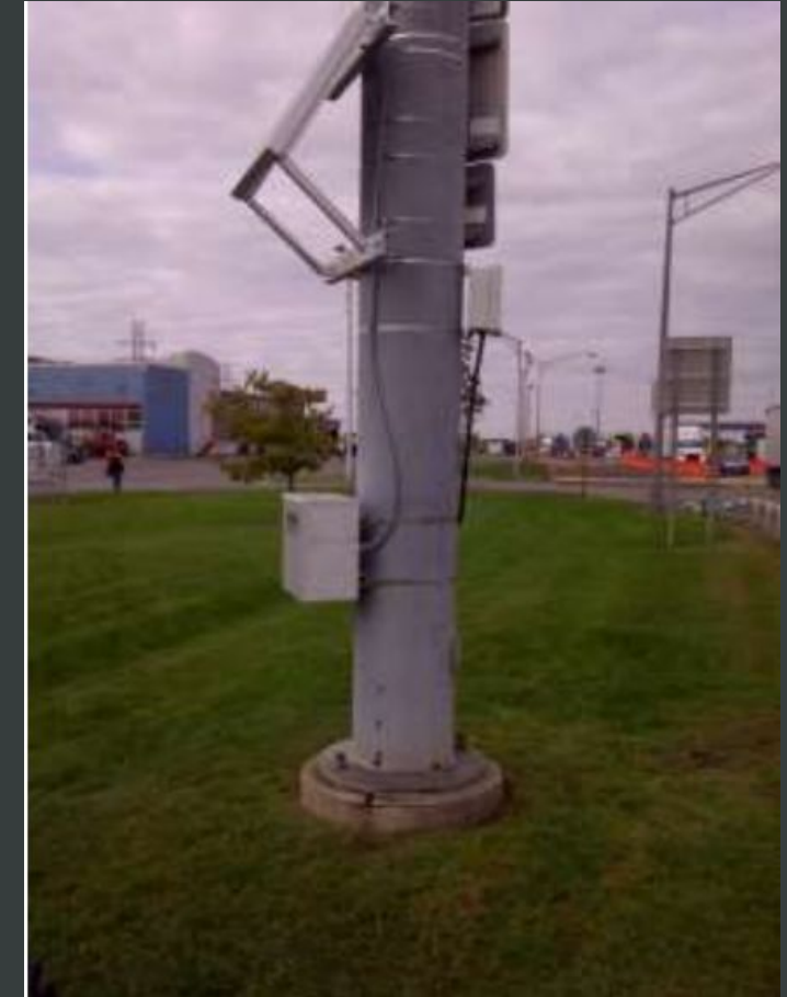
Bluetooth Reader in Solar Powered Configuration (per TPA North America)
